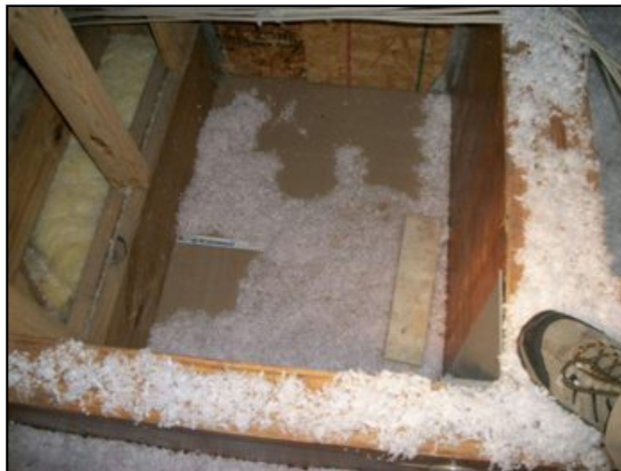
36. Missing insulation
