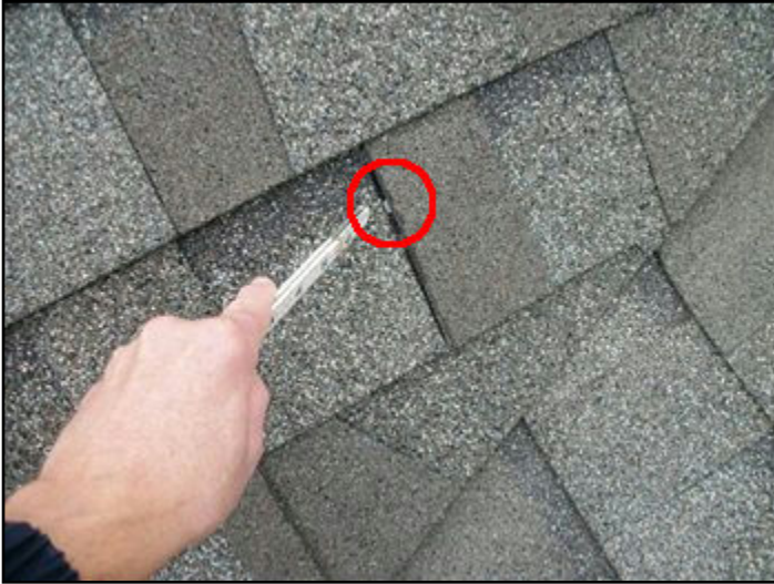
10. Exposed fastener-valley near side porch
