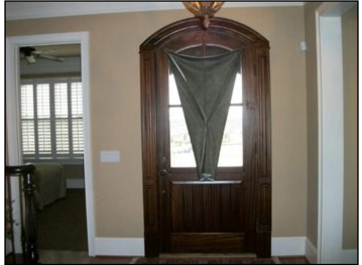
46. Front door facing west
